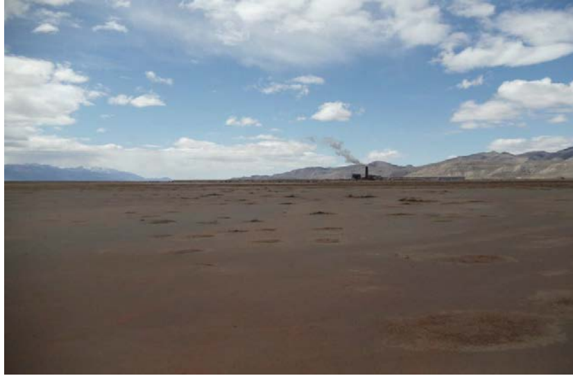
NE Waste Lagoon (Inactive)
