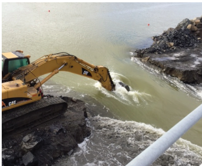
Removal of the southern access road to open the bridge, December 1, 2016 – photo courtesy of HDR Engineering
