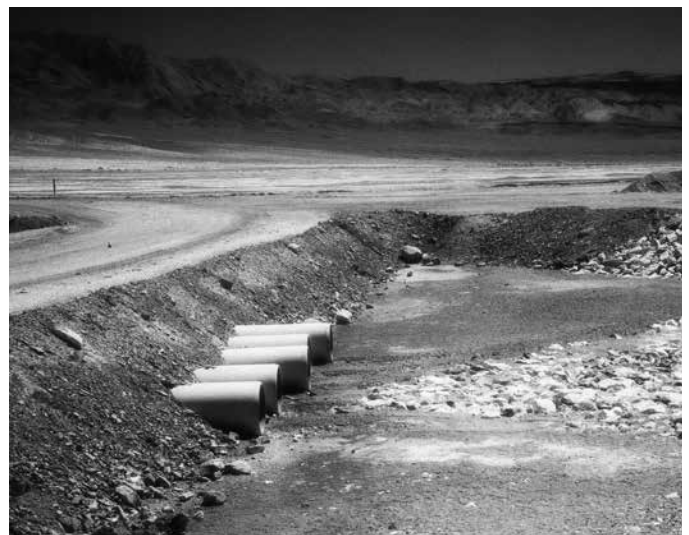
Numerous pipes carry fresh water from the Los Angeles Aqueduct to Owens Lake where it is distributed as a dust control method photo courtesy of Rosalie Winard
